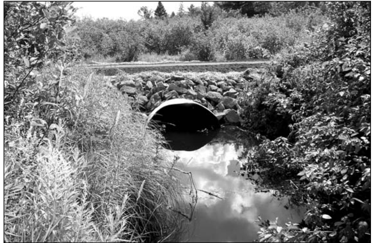
Repaired culvert at Montreal Creek and County Line Road.
