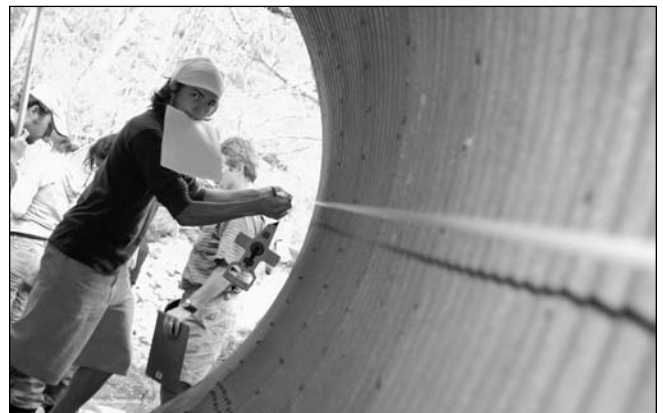
Matt Velie measures a culvert.
